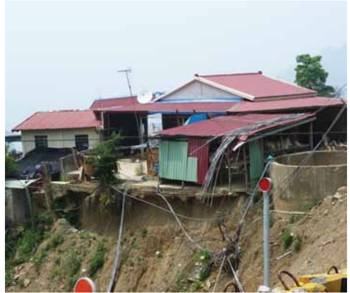
Above, an earthquake causes a major landslide. Photo courtesy Hsio-Ying Lo.
